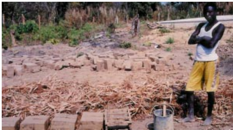
Anthill soil is mixed with sand and dried to make blocks, which are then fired to result in hard bricks.
